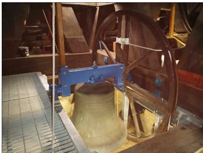
The flat 6th ready in its new home under the bourdon bell
