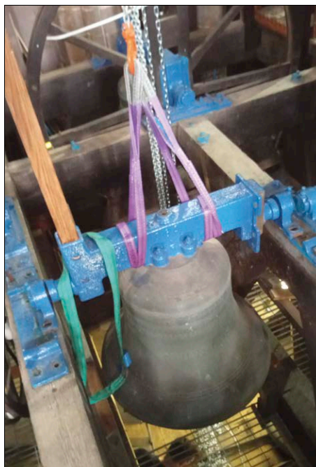
The 5# lowered into the old 6b pit
