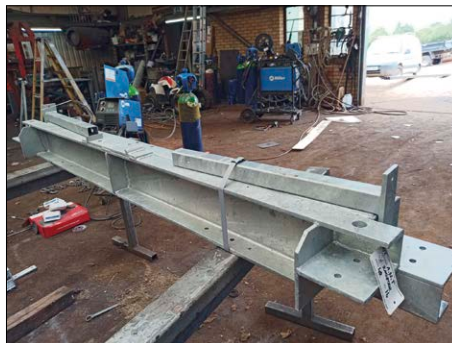
Some of the framework ready for assembly
