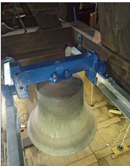
The flat 6th sitting on the new framework, 15th September
